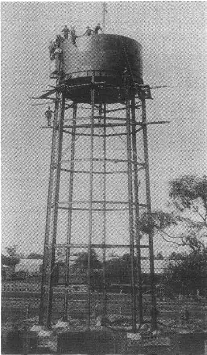
Water Tower under construction, 1910
