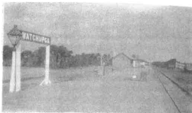
Watchupga station about 1935. The lamp near the station sign in addition to providing station lighting, was used to "flag" down trains during the hours of darkness using a red glass overlap. Flags were used in daylight hours. Kinnabulla had a similar set up.
