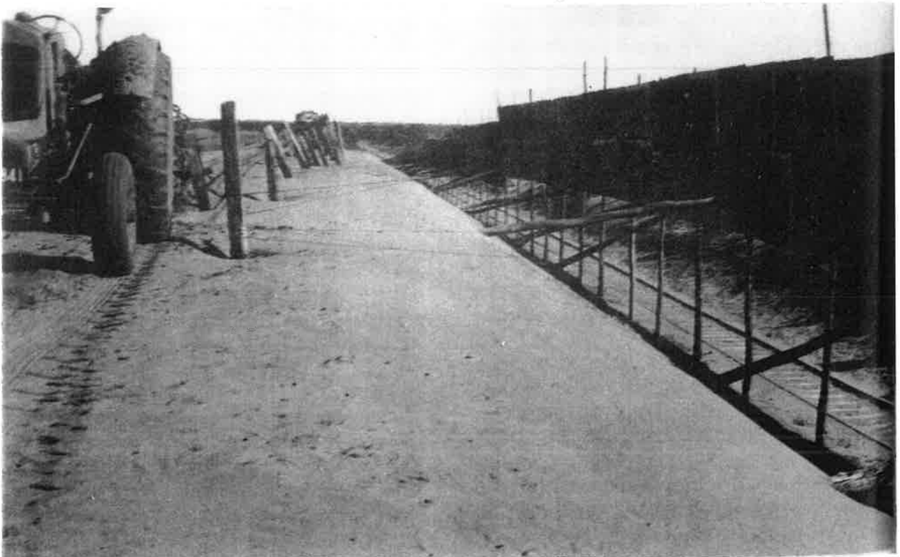
Wind chute at Light's Hill north of Curyo in 1944. The chutes helped to keep the track clear of sand.
