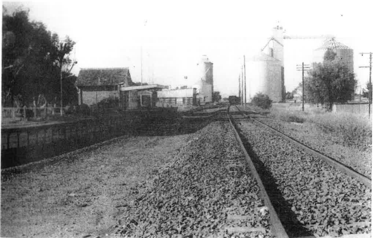
View of Birchip yard with Number one road adjacent to the platform and silo inclined 1:250 gradient outloading loop on the right. Photo taken 20th January 1993.
