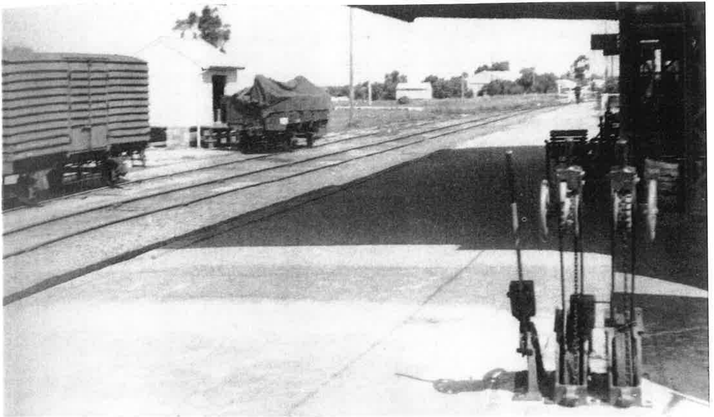
Another view of the Birchip station showing the small goods shed on the eastern side of the tracks. Signal setting levers may be seen on the platform in the foreground. Photo taken October 1975.
